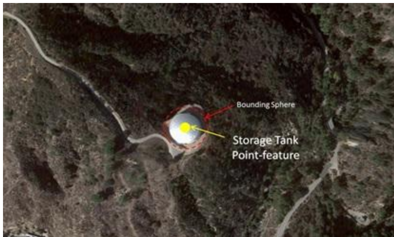
Figure 5- 12: Storage Tank Point-Feature
